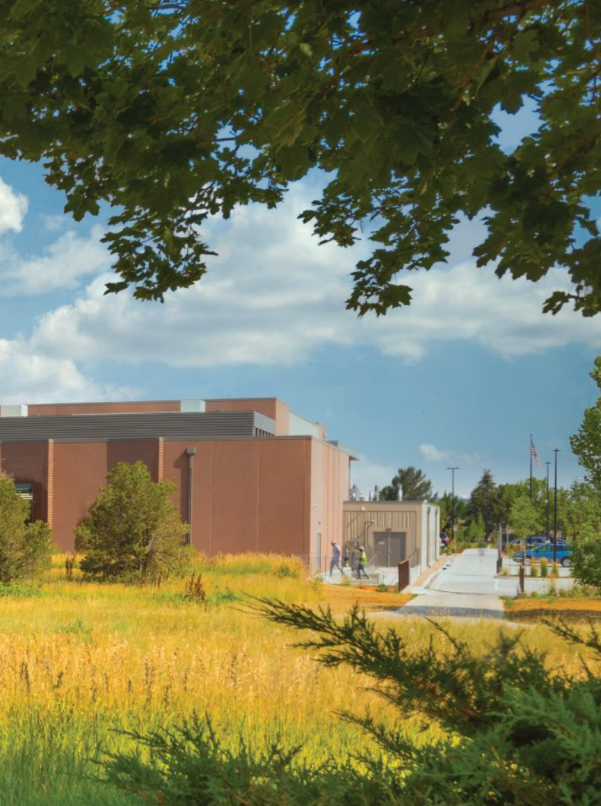
On the north side of the site, the community center is only 10 ft away from protected wetlands. The project team took great care not to disturb any protected areas. Photo: WELLS.
